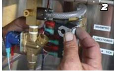
After the Nut is off, pull off the coil.
