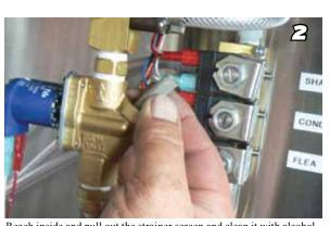
Reach inside and pull out the strainer screen and clean it with alcohol and water. Replace if worn.
