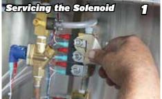
First be sure the Power is OFF or you will blow the coil. Start at the top of the block, working your way down, one solenoid at a time. Unscrew the nut.
