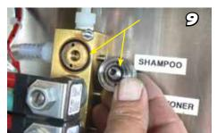
Check both O-rings for wear and replace if needed.
